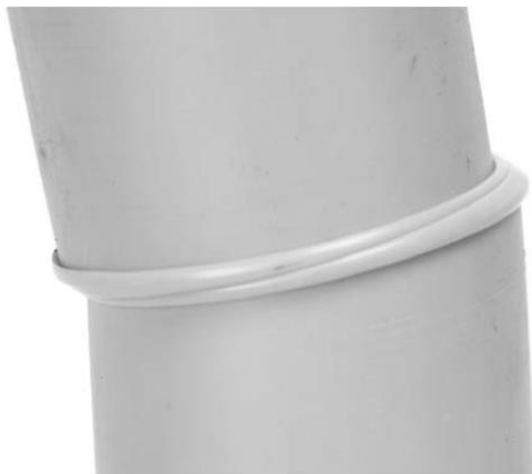
“high-low” pipe alignment. Visually mitered joint.
